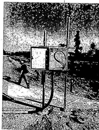
C. Telemetry unit mounted on poles set in concrete within augered holes, adjacent to existing concrete pad; arrows show extent of new concrete
