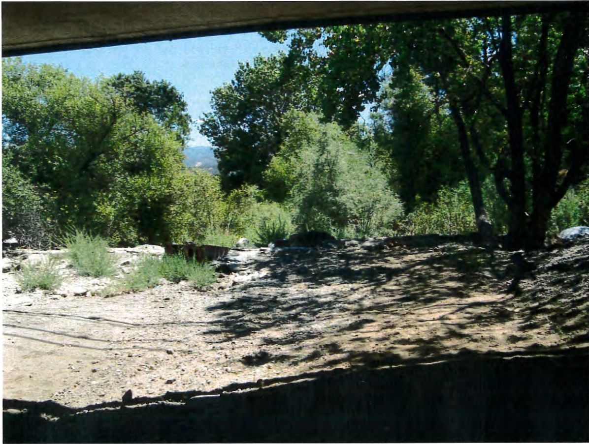
Figure 6: Looking downstream at the channel and grade control structure. The overbank areas are heavily vegetated with relatively high manning “n” values
