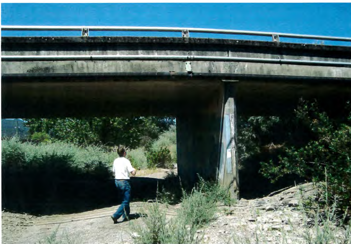
Figure 12: Looking upstream at the existing bridge
