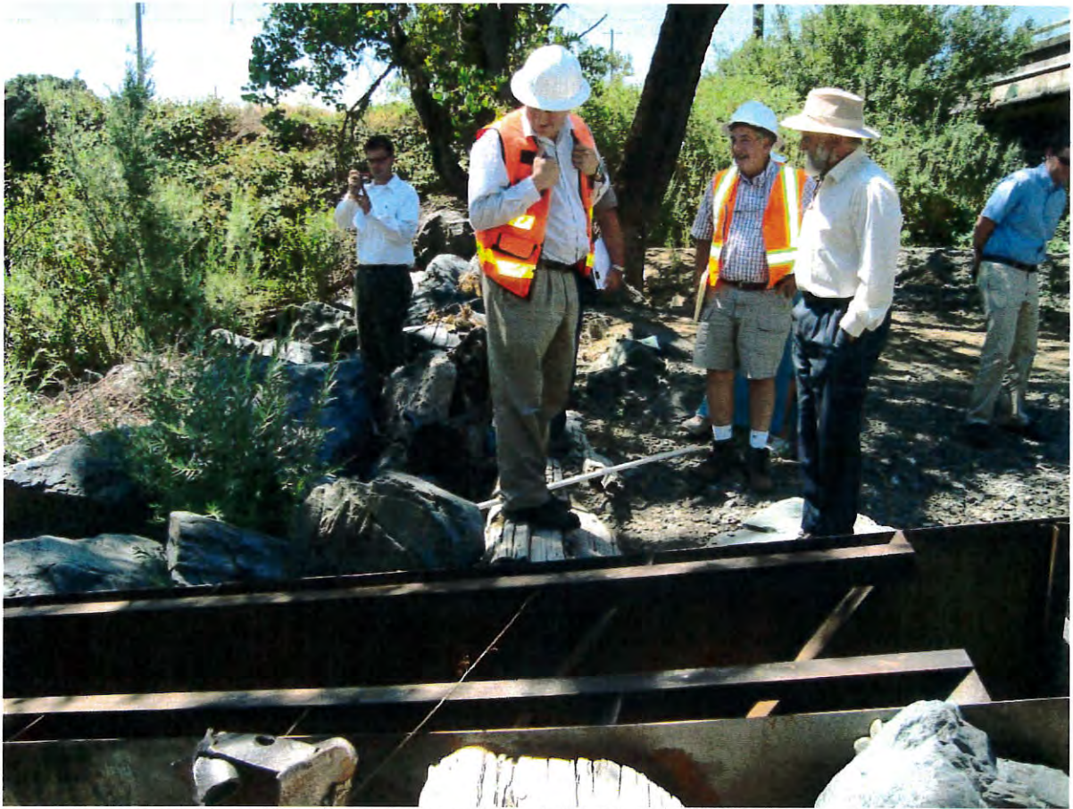
Figure 15: Looking at the grade control structure during the July 21, 2011 Field Review (photo by Avila)
