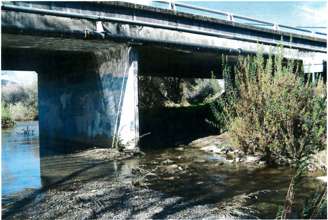
Figure 2: (top) Picture facing west looking upstream at one of the existing bridge piers.
